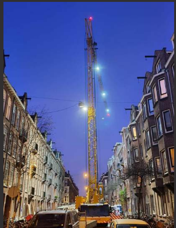
Snapper on mobile light tower
